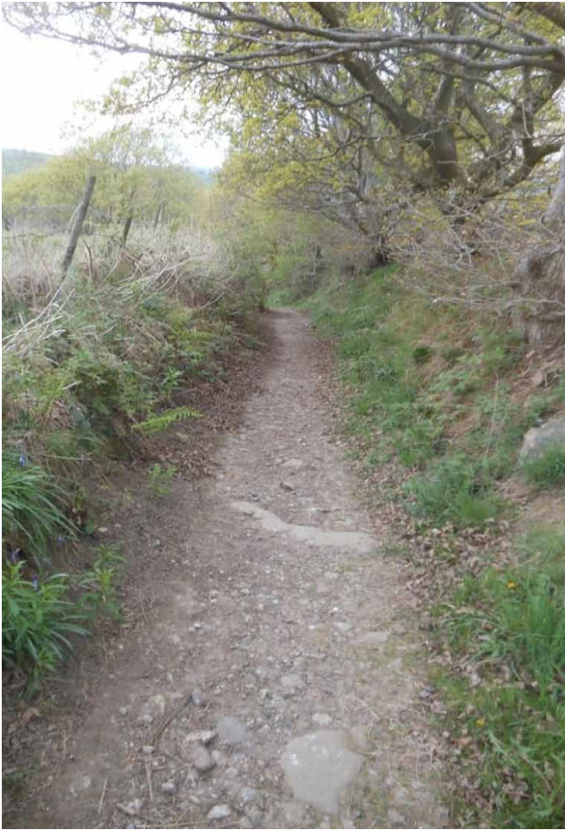
The Worrall path – pilot project. A hollow way, showing a compacted stone surface. The features shown here are typical of an old highway and are the type of thing that volunteers will be looking for when they survey routes. Photo credit: Melanie Fitzgerald
