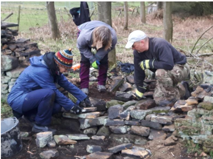
Narelle Willis, Assistant Ranger for SLLP, starting to learn the basic techniques of Dry Stone Walling before beginning the formal LANTRA Level 1 Dry Stone Training.
